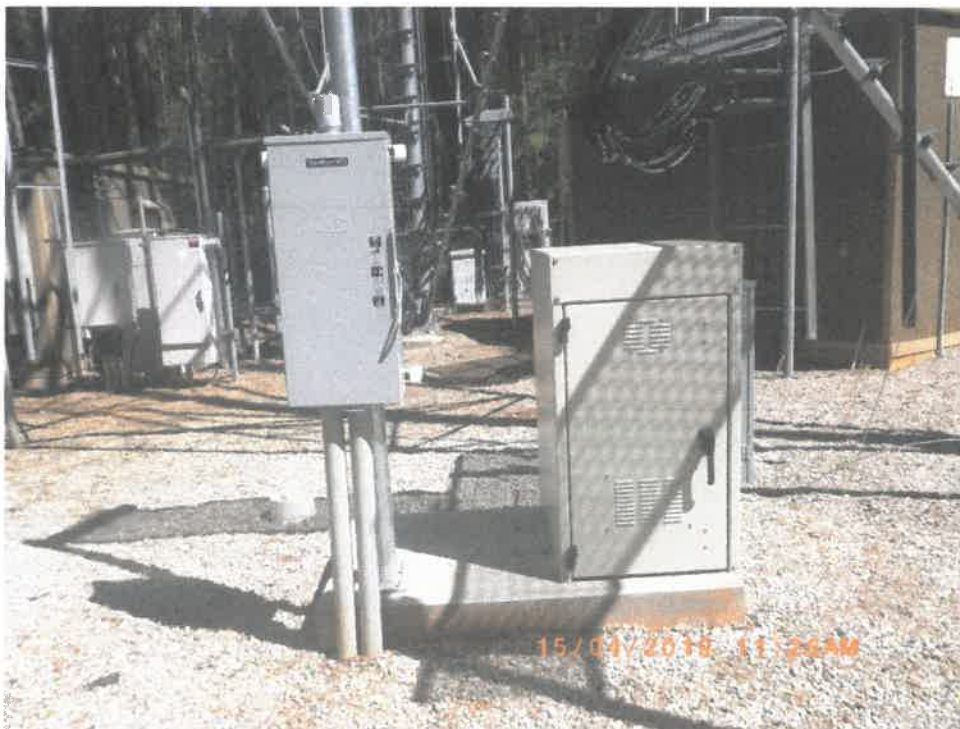
B.2 – Visual representation of system installation at water tower base. Cabling will be run up the side of the tower, connecting the tower base installation to the tower roof installation.
